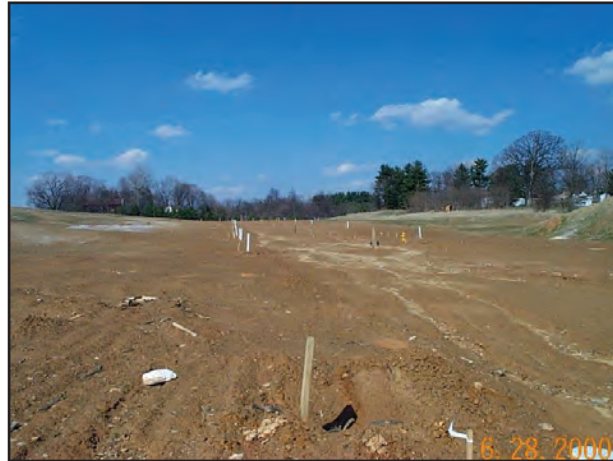
During construction, vegetation is cleared and the development site is graded to prepare for construction. With the trees and topsoil removed, soils are particularly susceptible to erosion. Photo Copyright 2000, Center for Watershed Protection
