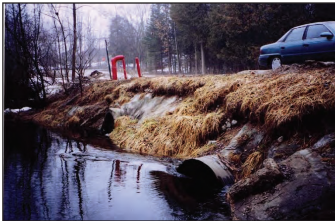
Road stream crossings, like this one shown on the Rapid River in Kalkaska County, are a common source of sediment to streams. Photo courtesy of the Kalkaska Conservation District
