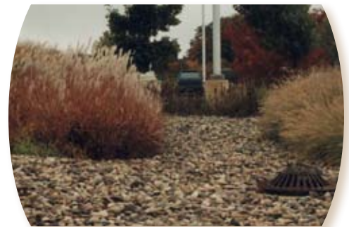
Infiltration Basin – Photo Courtesy of Don Tilton
