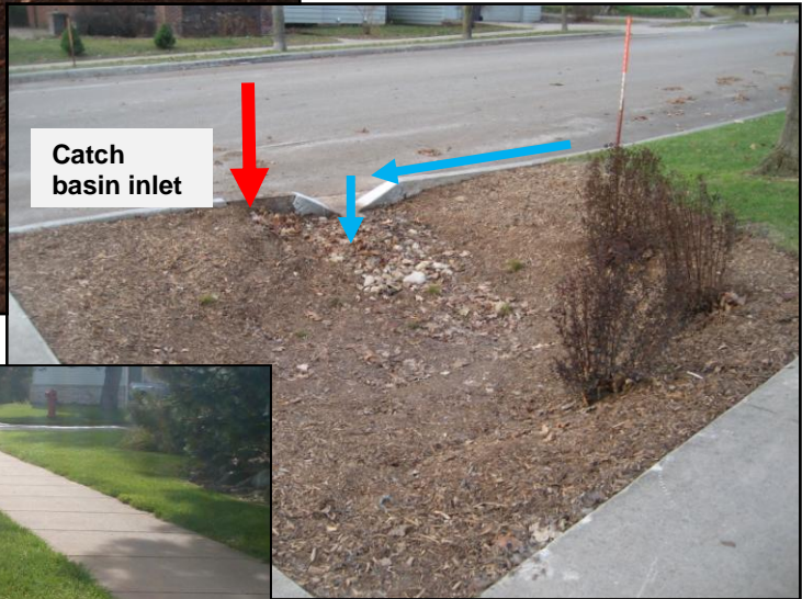
Examples of rain gardens installed in Suttons Bay where water is collected via curb and gutters into rain gardens. As rain gardens fill up, water will start bypassing the garden and go to existing catch basins.
