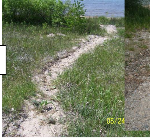
Erosion at Bunker Hill road
