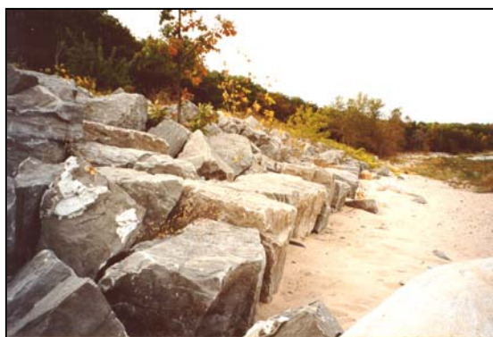
Example of shore hardening using large rock rip-rap.
