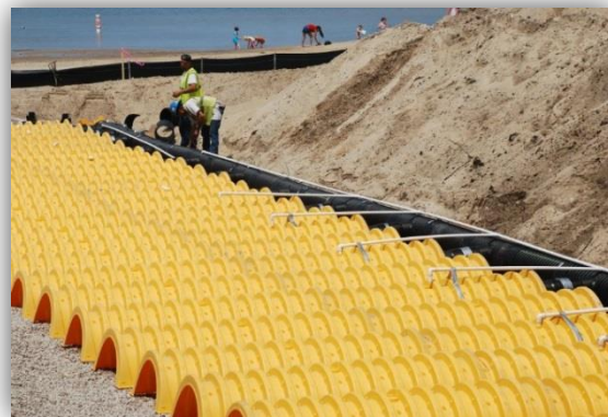
Underground infiltration trench at Bryant Park, Traverse City Photo courtesy of: The Watershed Center Grand Traverse Bay
